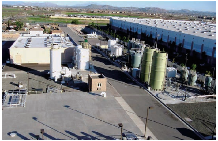
View of the Chino I Desalter facility.
